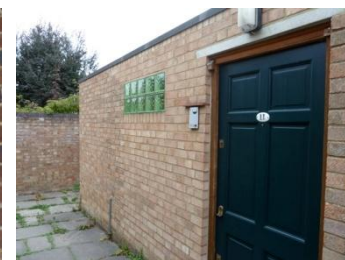
Glass blocks in nearby rd
