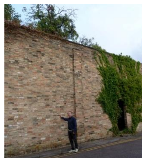
High wall in adjacent street
