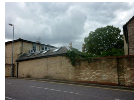
Even higher wall adjacent buildings on West side of Fitzroy Street
