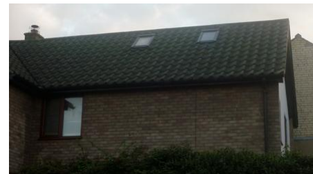
Existing rooflights at 68 Maids Causeway
