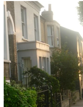
Flat roof projection at 54 Maids Causeway
